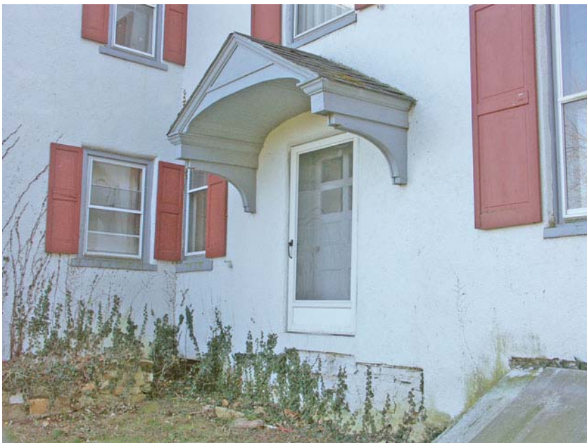
Photo 5. View of the arcuated hood over the back door. Note also the markings under the door where the porch once stood.
