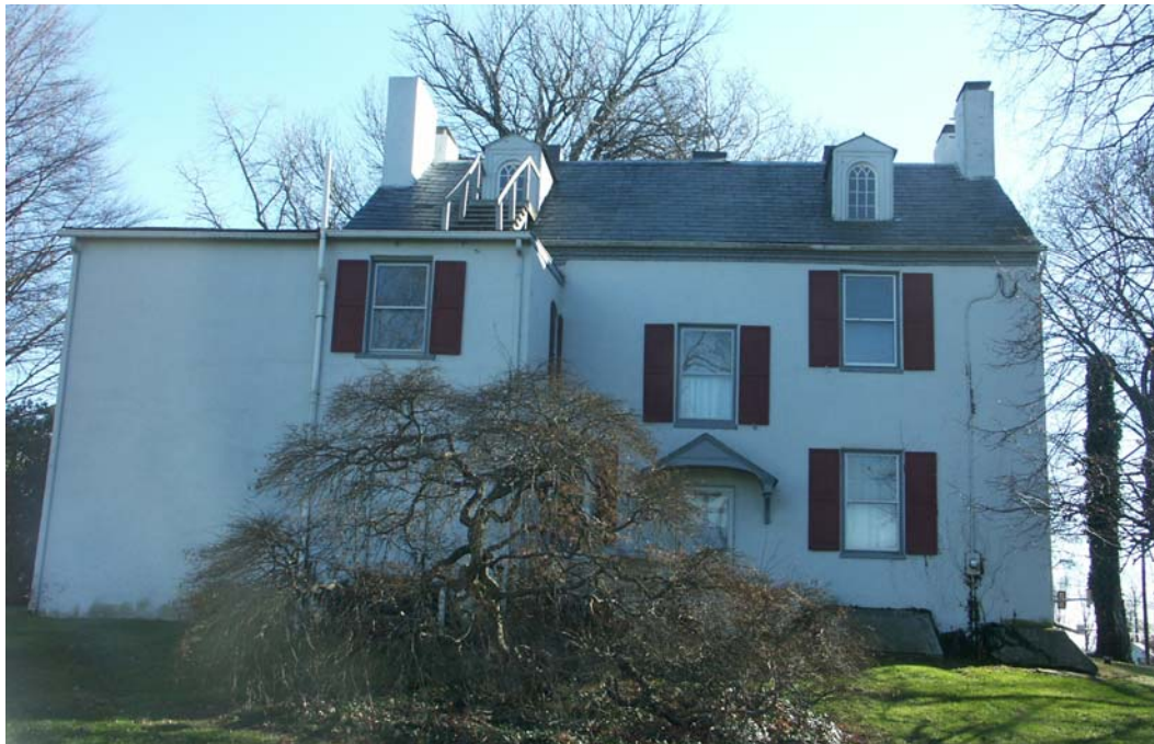
Photo 4. North elevation, showing the rear addition (left) and main block (right).
