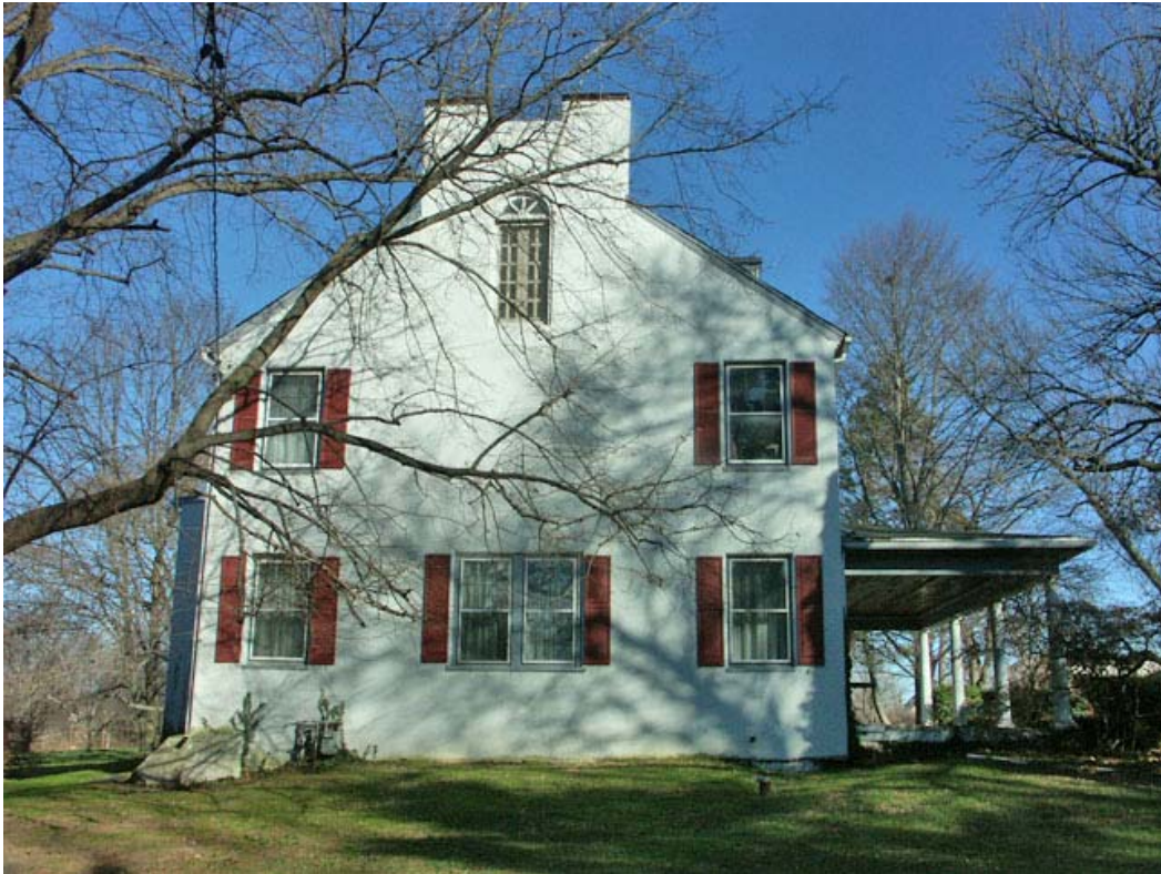
Photo 3. West end of Main Block. Note the Colonial Revival style French door at the attic level.
