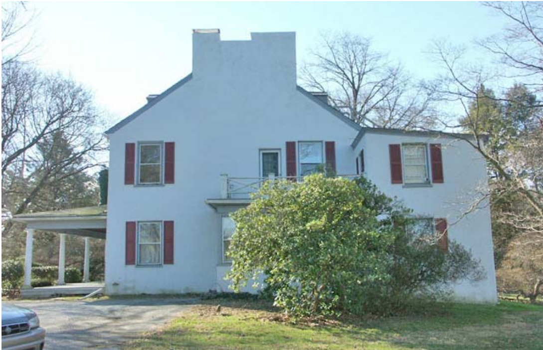
Photo 6. East elevation. Visible sections are the main block (center), enclosed porch (behind shrub), and rear addition (right).
